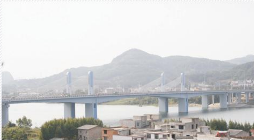
Sanmenjiang Bridge in Liuzhou
